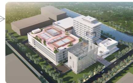
昆山智慧工厂(在建) Kunshan SMART Factory 40,000 m 2 (Under Construction)
